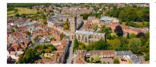
The tower rises 174 feet to the pinnacles and, following significant deterioration, is currently subject to substantial and costly repairs. The intention is to carry out works to preserve and make safe as much of the original stonework as possible.
